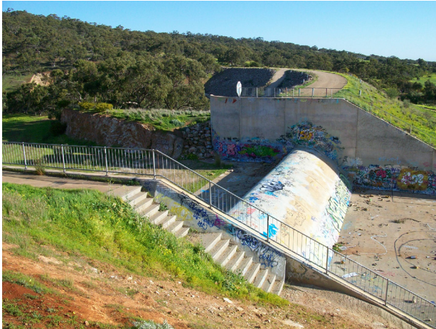
Dam in Cobblers Creek Recreation Park
