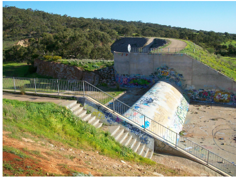
Dam in Cobblers Creek Recreation Park
