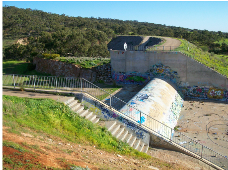
Dam in Cobblers Creek Recreation Park
