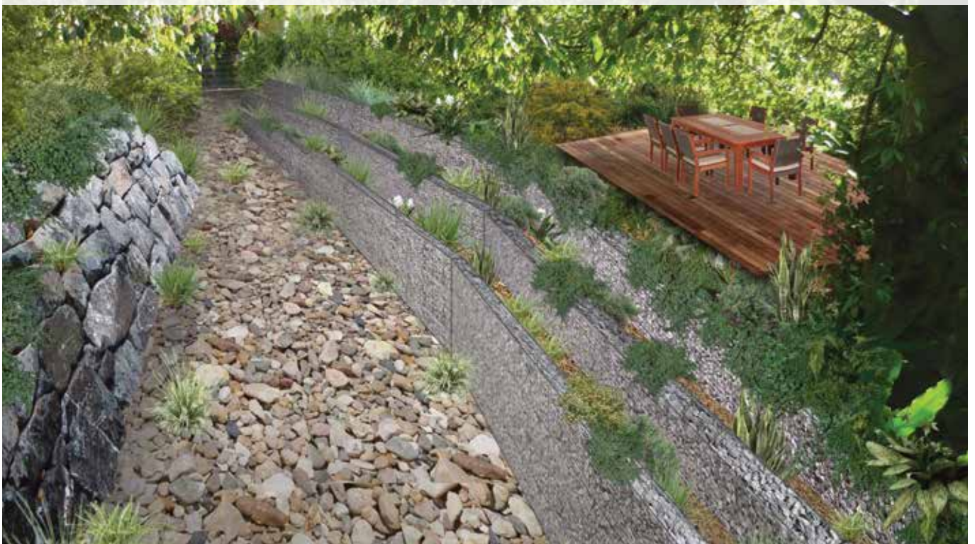
After – using gabions (rock filled wire baskets)
